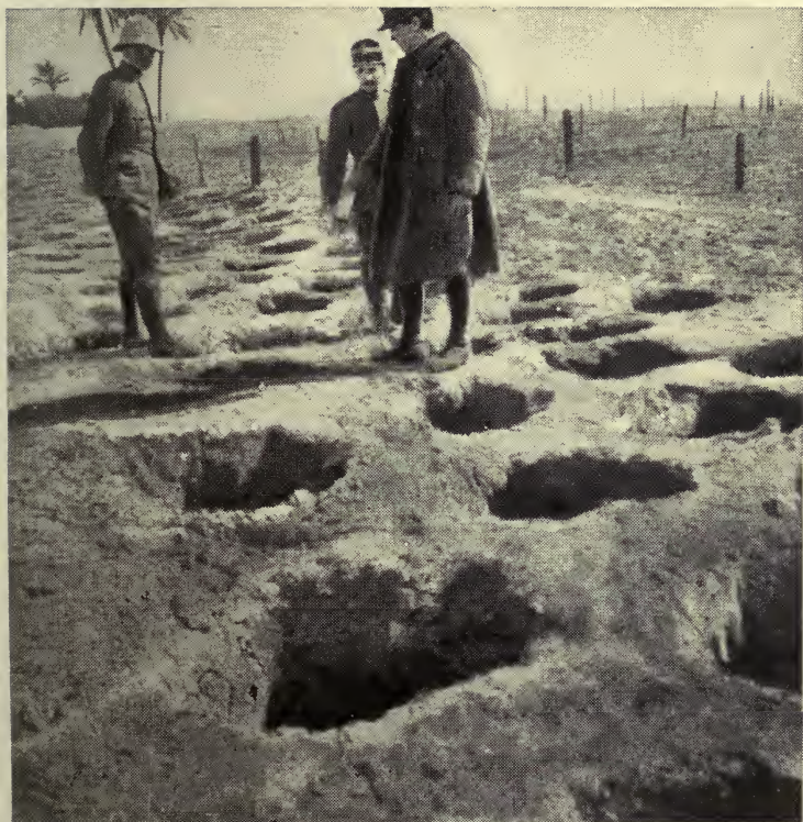
TRAP-HOLES AND BARBED-WIRE ENTANGLEMENTS WHICH PROTECT THE ITALIAN TRENCHES
